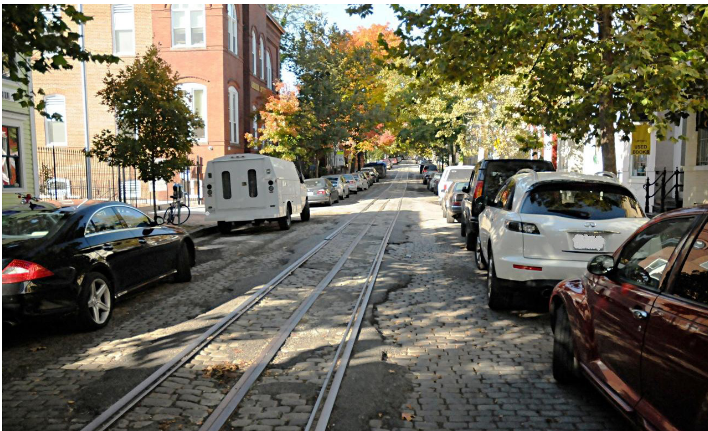
Many District streets are unique and require a tailored approach to rehabilitation
