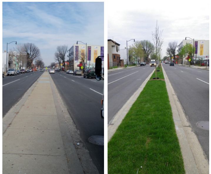
Green median renovation on Bladensburg Road NE
