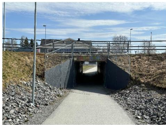
(d) Illustration of the other side of bridge - towards skolevegen
