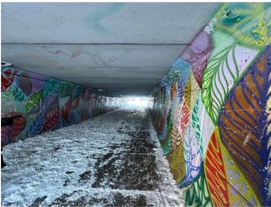
(c) Entrance of the tunnel for foot traffic
